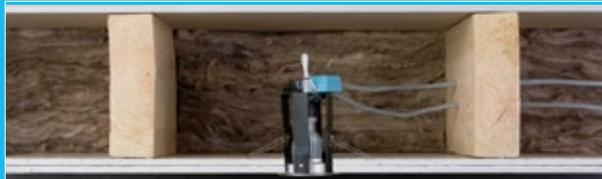
The ceiling is constructed with ceiling joists at 450mm spacings and a dual layer of 15mm plasterboard fixed to the underside of the joist.
