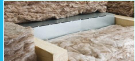
Note: iBox is not designed to provide a load bearing platform within a roof void.
