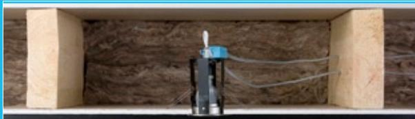
The ceiling is constructed with ceiling joists at 600mm spacings and a single layer of 12.5mm plasterboard fixed to the underside of the joist.
